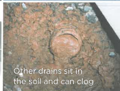
TYPICAL CLOGGED DRAINTILE
